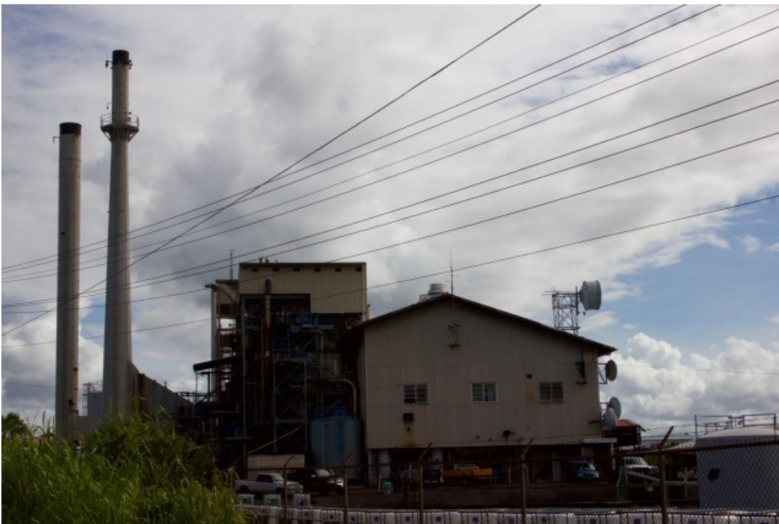
HELCO's Kanoelehua Hill generating station in Hilo.
